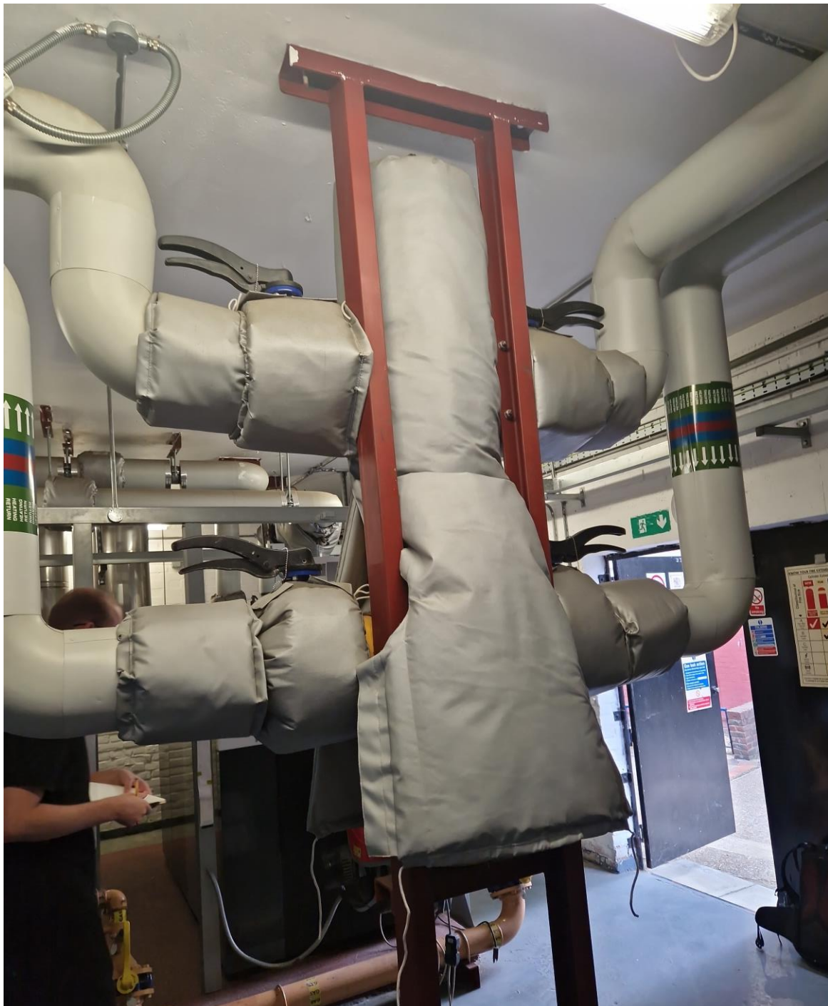
Figure 31: Combined low loss header and air/dirt separator
